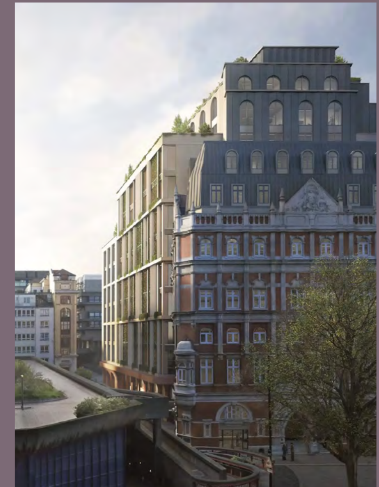
View showing the retained grade II listed facade Source: Planning Application DAS
