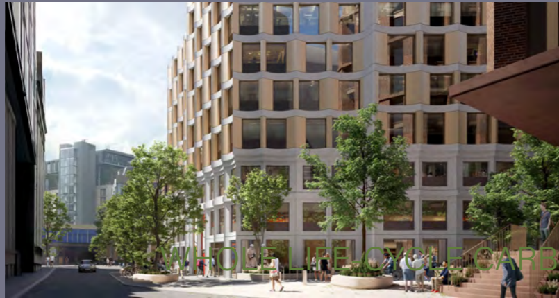
Ground floor view of 65 Crutched Friars Source: 65crutchedfriars.co.uk 2023
