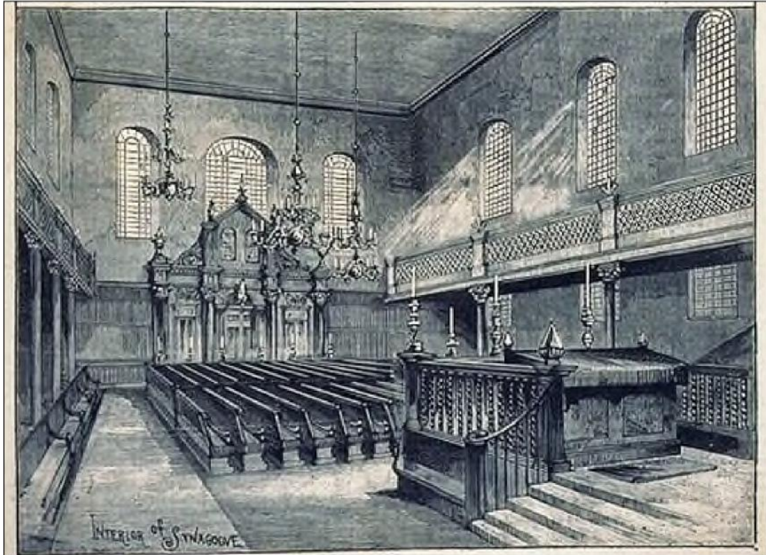
Bevis Marks Synagogue, 1891 - Showing light entering the building from its southeast
