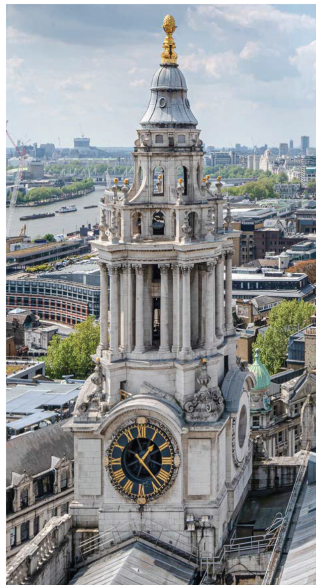
The SW Tower of St Paul’s Cathedral (picture credit: Historic England).
