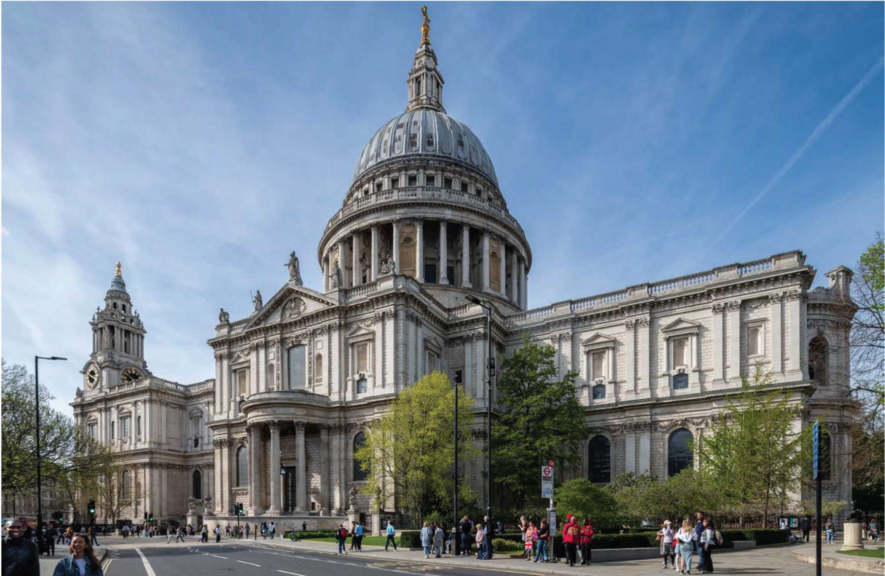
St Paul's dome from the south east where the plain base, the columned peristyle, the upper drum the dome itself and the crowning lantern can all be appreciated as the central crossing point of the design (picture credit: Historic England).
