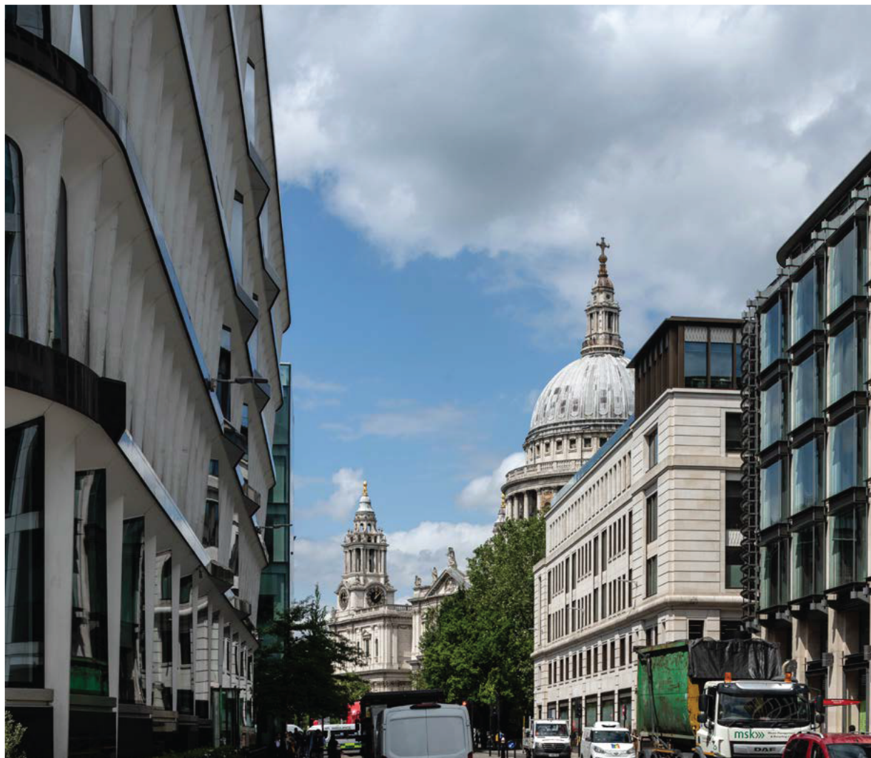
St Paul's from Cannon Street to the east at the junction with Queen Victoria Street. The bronze clad penthouse element on 31 Cannon Street in the foreground collides with and obscures part of the important silhouette and form of the dome of the Cathedral. Photograph by the author 2023 (picture credit: copyright Historic England).
