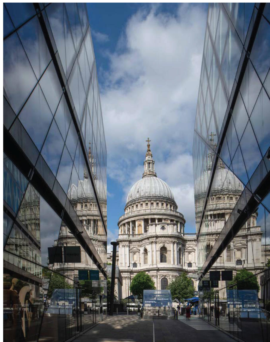
East end of St Paul's Cathedral seen from within New Change (picture credit: copyright Historic England).
