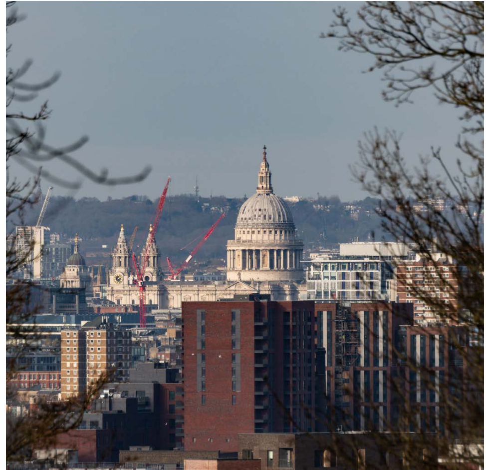
Detail of central element of the view showing the impact of foreground development upon an ability to appreciate the architectural composition of the Cathedral and undermining its intended dominance (© Historic England Archive)
