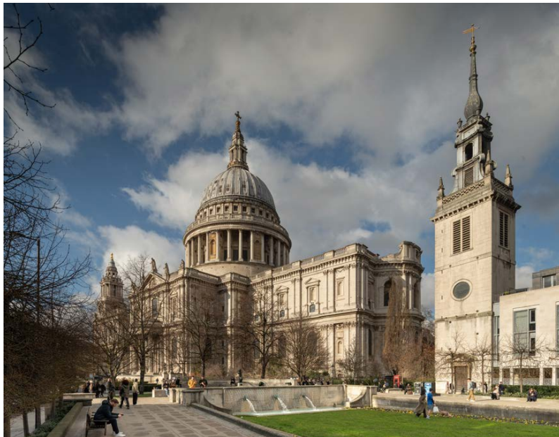
St Paul's Close setting from the South-East (© Historic England Archive)
