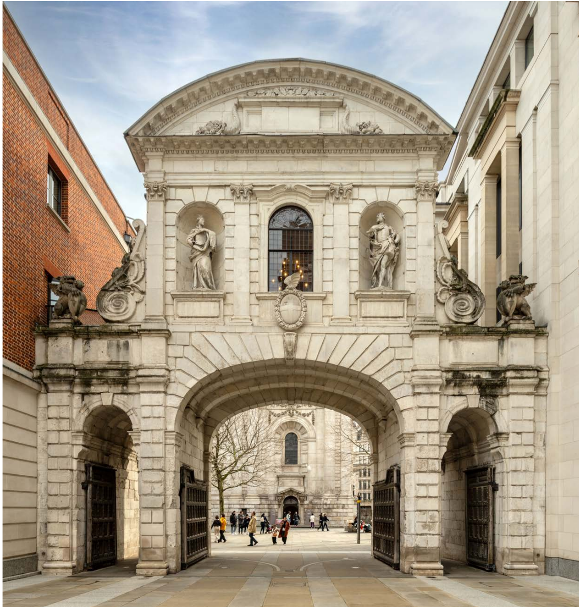
View under Temple Bar towards the north transept of the Cathedral (© Historic England Archive)
