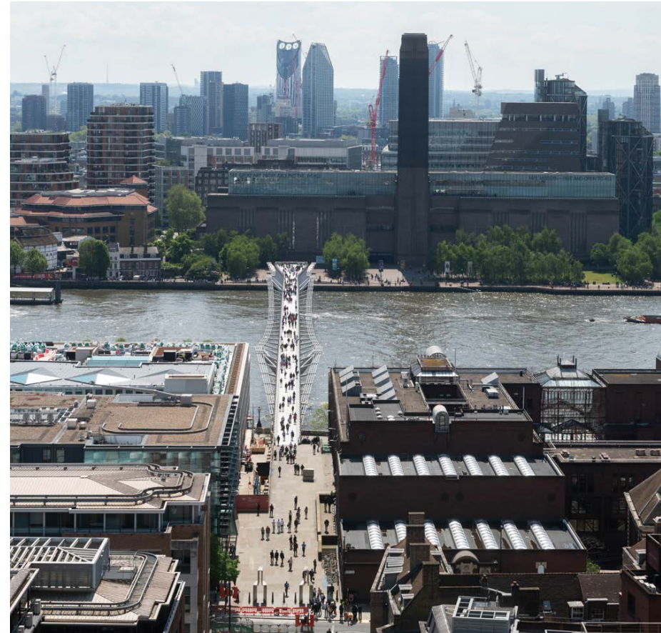
The Millennium Bridge and St Paul's Hill from the Stone Gallery linking with Tate Modern and The Globe on the South Bank; the most popular pedestrian visitor route to the Cathedral (© Historic England Archive)
