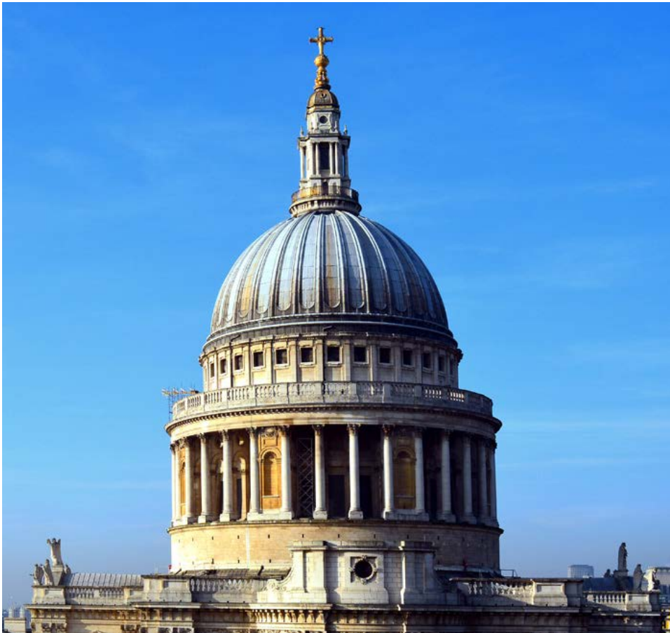
St Paul's Cathedral dome, balustrade and statuary from the roof terrace of One New Change
