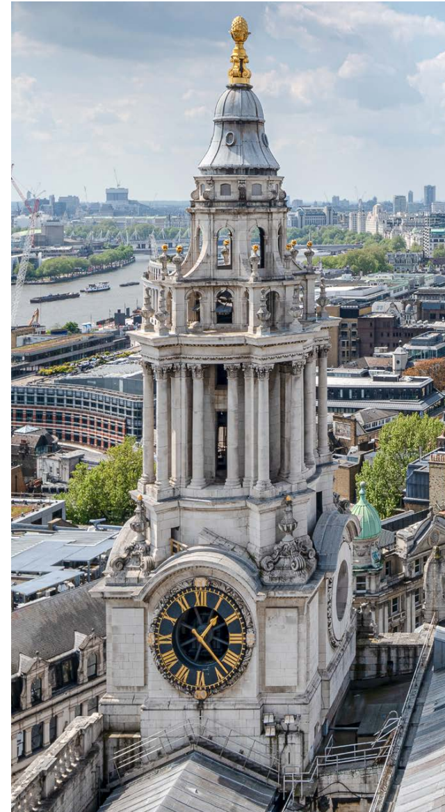
The South West Tower of St Paul's Cathedral (© Historic England Archive)
