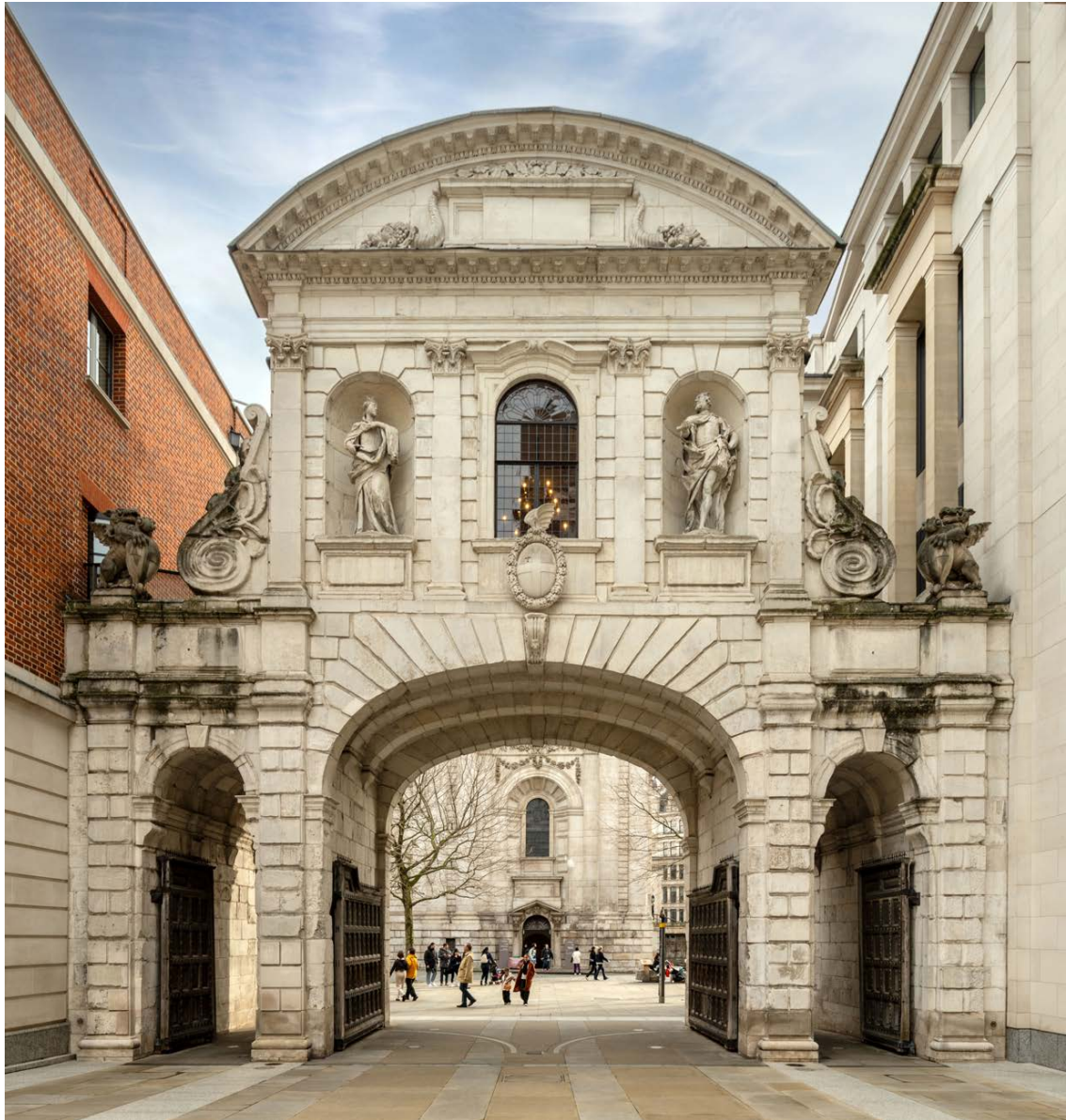
View under Temple Bar towards the north transept of the Cathedral (© Historic England Archive)
