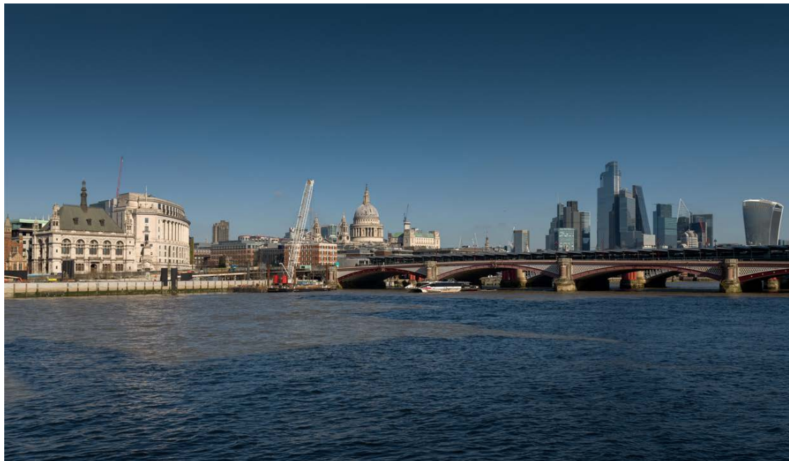
Views towards the Cathedral from the Queen's Walk adjacent to the Oxo Tower (© Historic England Archive)
