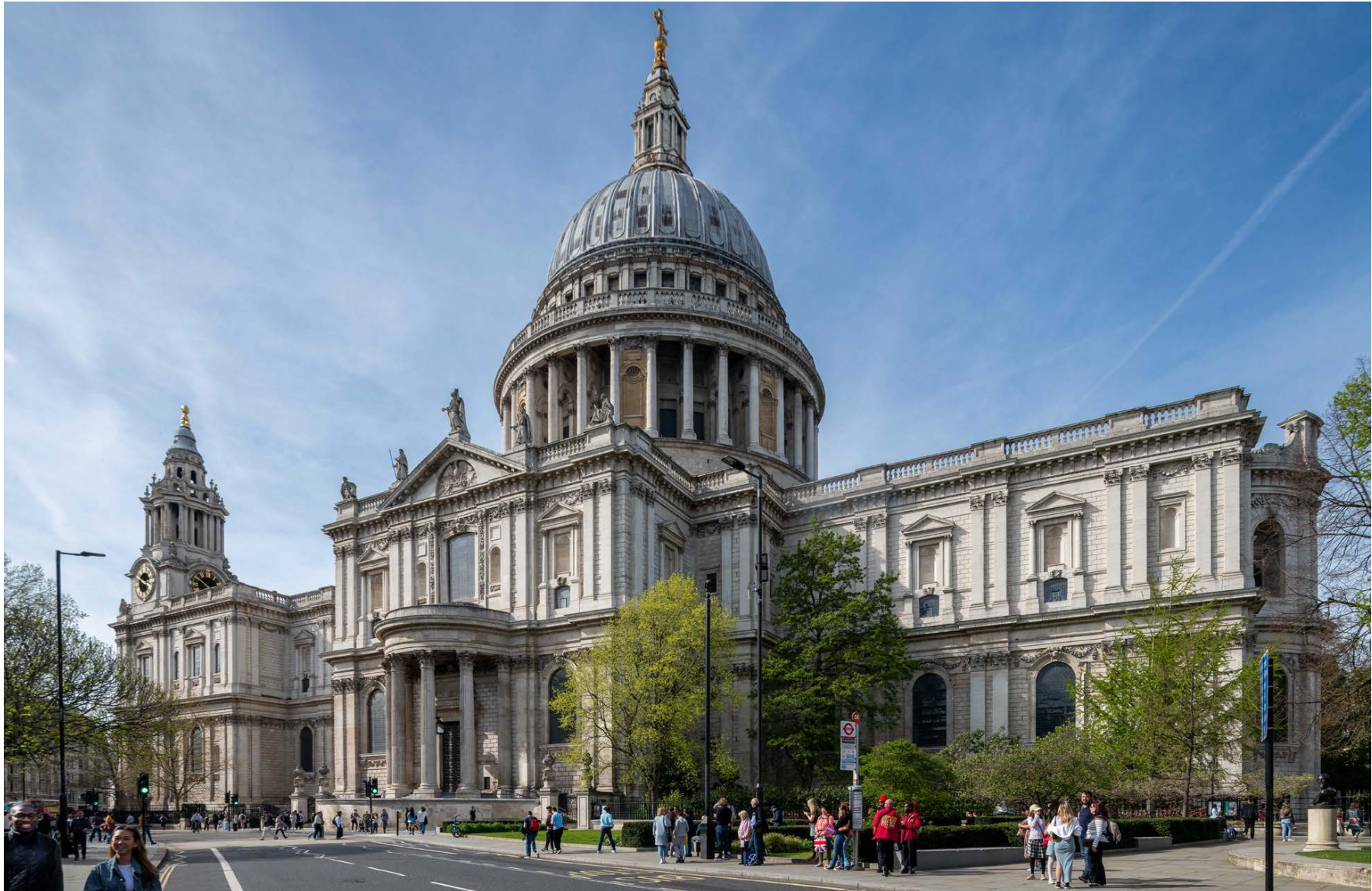
St Paul's dome from the south east where the plain base, the columned peristyle, the upper drum the dome itself and the crowning lantern can all be appreciated as the central crossing point of the design (© Historic England Archive)
