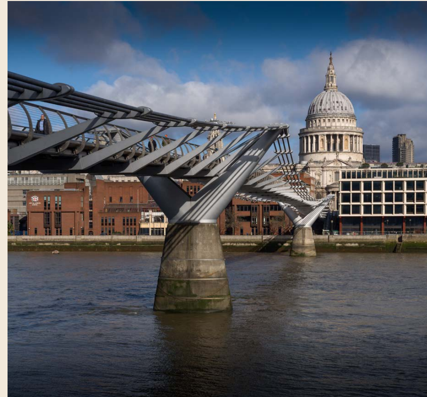
St Paul's from the South Bank by Tate Modern and the Millennium Bridge providing an elevated pedestrian route across the river and aligned on the south transept of the Cathedral (© Historic England Archive)
