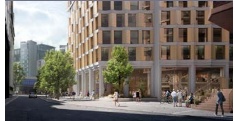
Ground floor view of 65 Crutched Friar. Source: 65crutchedfriars.co.uk 2023
