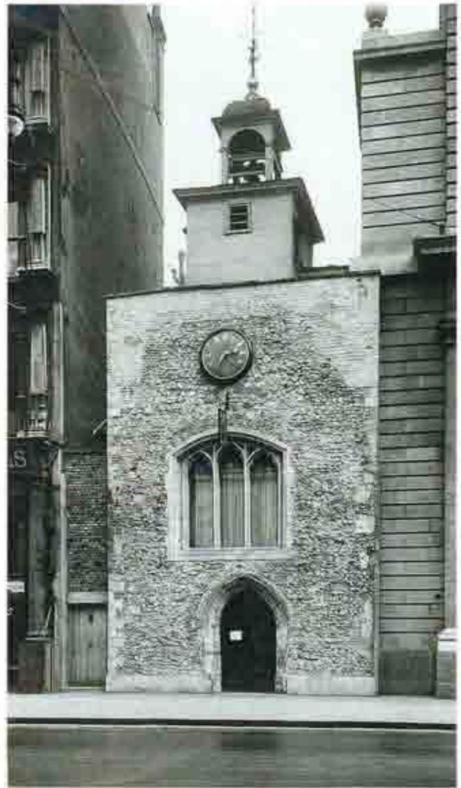
St. Ethelburga's after demolition of shops 1932
