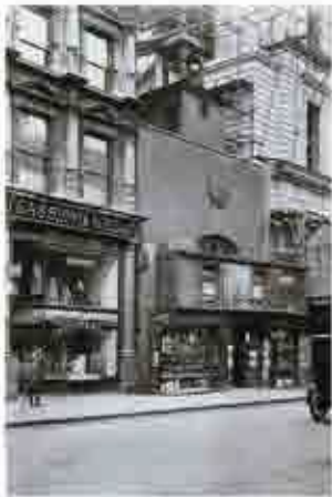
St. Ethelburga's before demolition of shops
