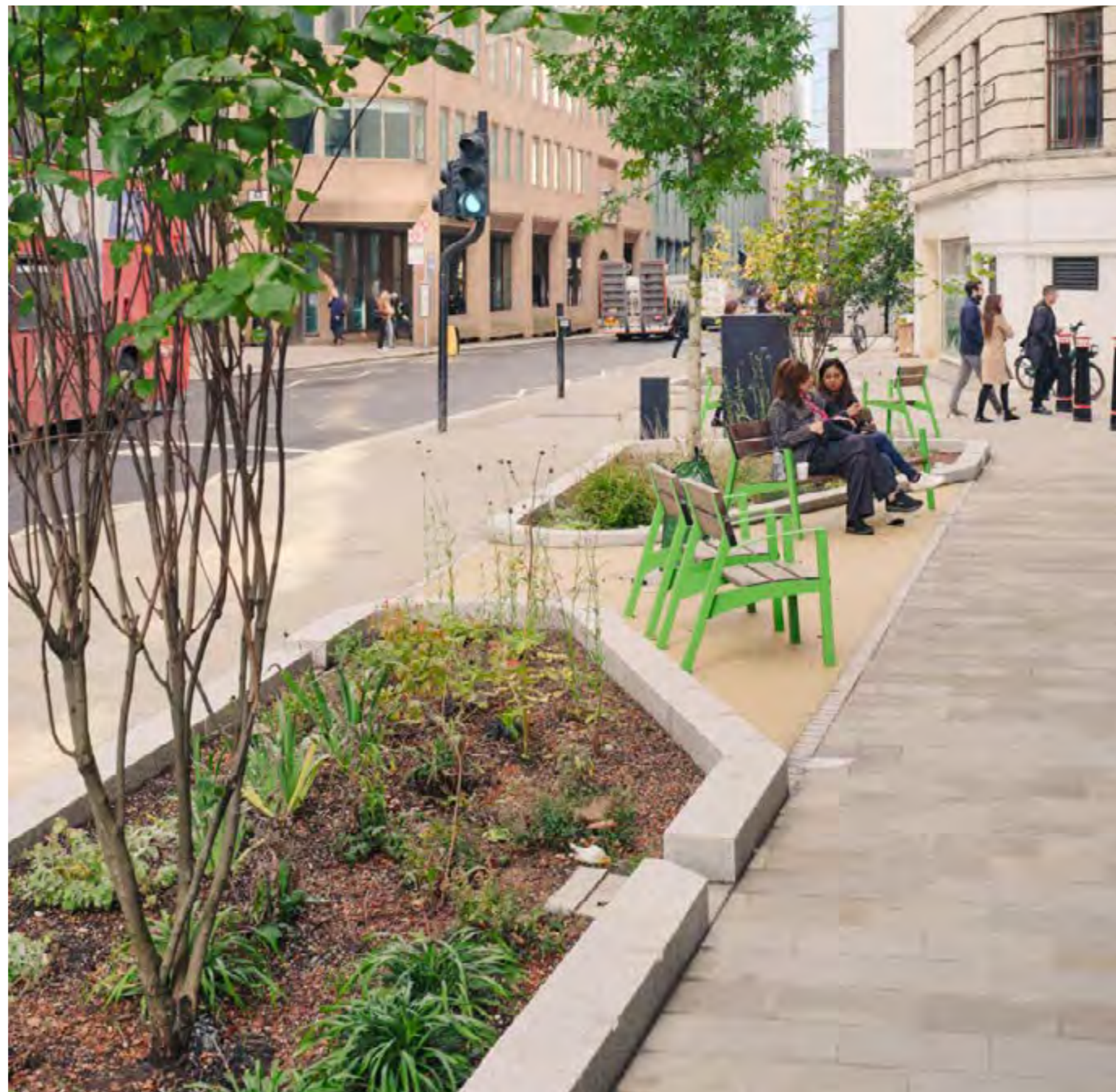
Bevis Marks Sustainable Drainage System schemes (SuDS)
